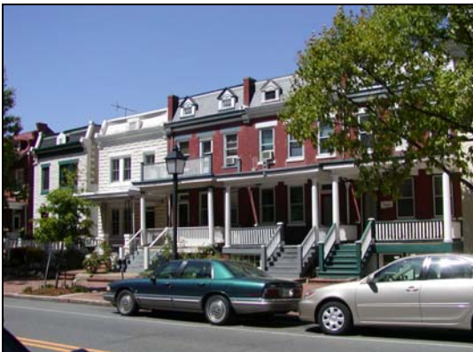
Residential townhomes with primary entrances to the street
