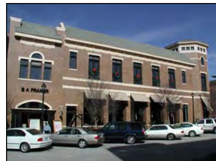
Vertically oriented windows with emphasis on corners and entrances.
