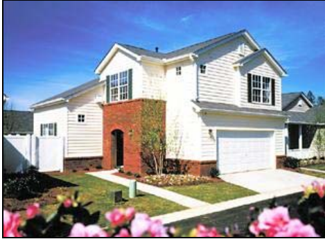
Residential building with garage in line with the front façade – not permitted
