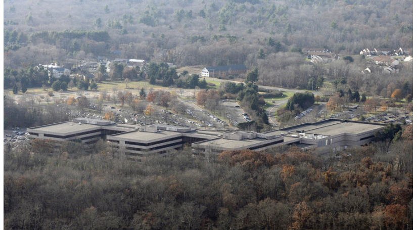
The Hartford's sprawling campus in Simsbury will be demolished. This photograph is the back side of the campus as seen from Talcott Mountain near Heublein Tower. (Hartford Courant File Photo)
